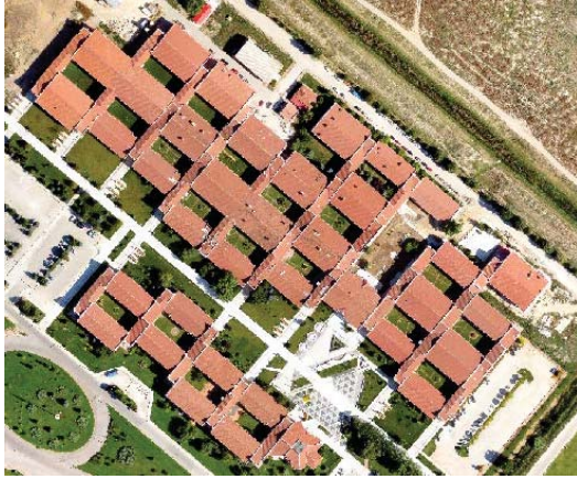
Fig.1. Orthoimage of Engineering Faculty İki Eylül Campus.
