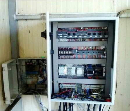
**Fig. 6.** Photograph of the board next to the PLC cabinet of the pilot sun-tracking system
